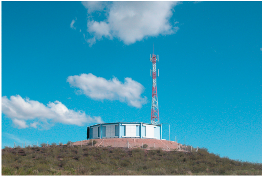
Figure 10: A picture of the FD building with closed shutters, from [2].
